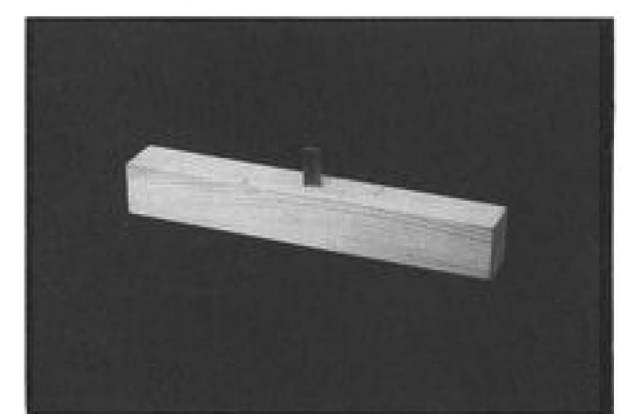
3 The splice is completed by locking it with a key.
