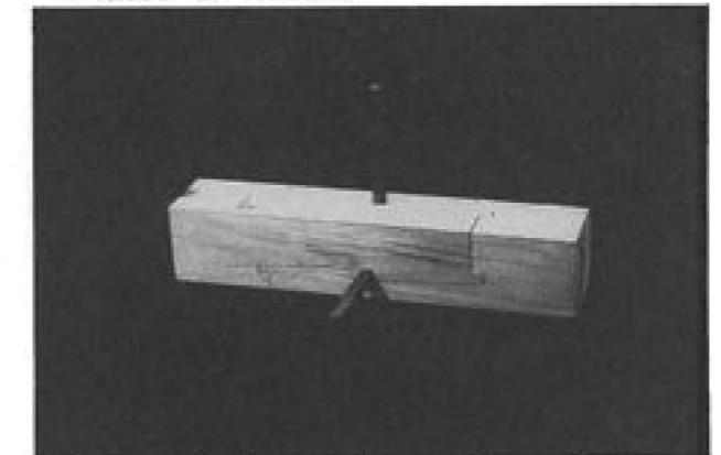
④ The splice is completed by inserting two draw pins.
