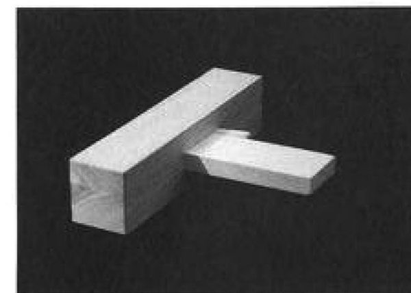
④ The joint is completed by driving in the wedge.
