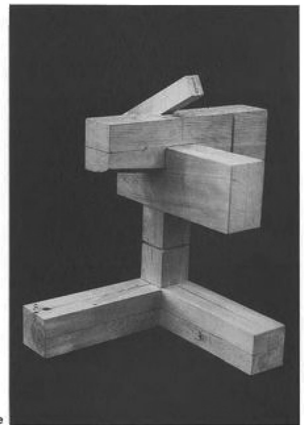
⑤ The rafter sits on top of the eave girder.
